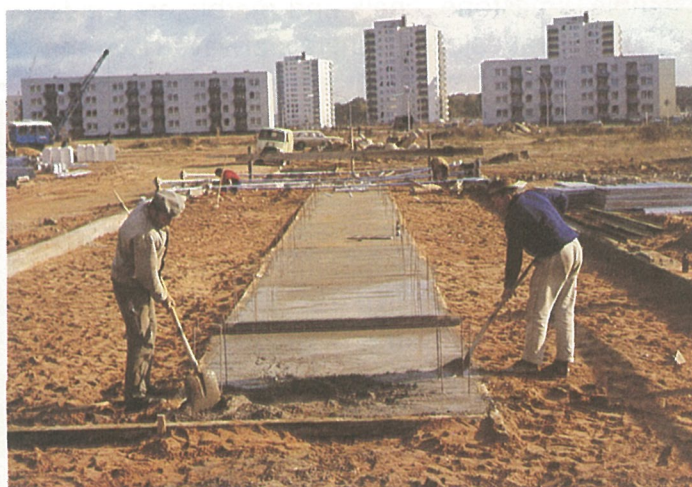
Above: Using concrete to make strong foundations.
