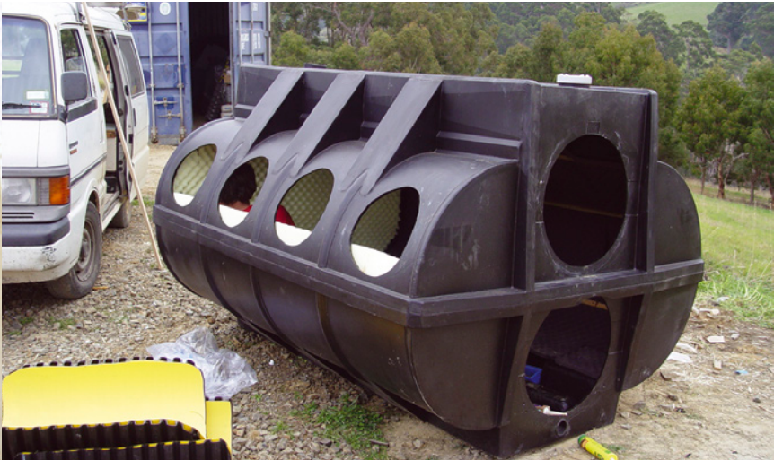
Bottom left: The straw bale rendering is probably the hardest aspect of straw bale construction. Below: The passive air-conditioning system incorporated a modified septic tank, buried underground, lined with deadening material.
